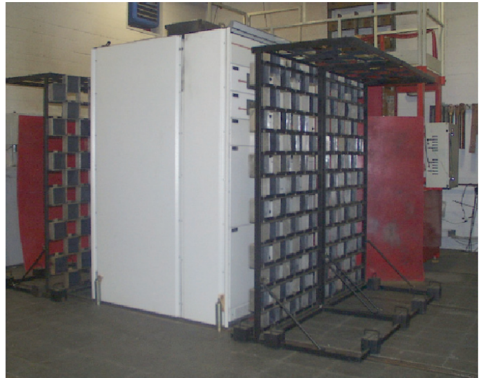
Switchboard under test according to IEC/TR 61641
