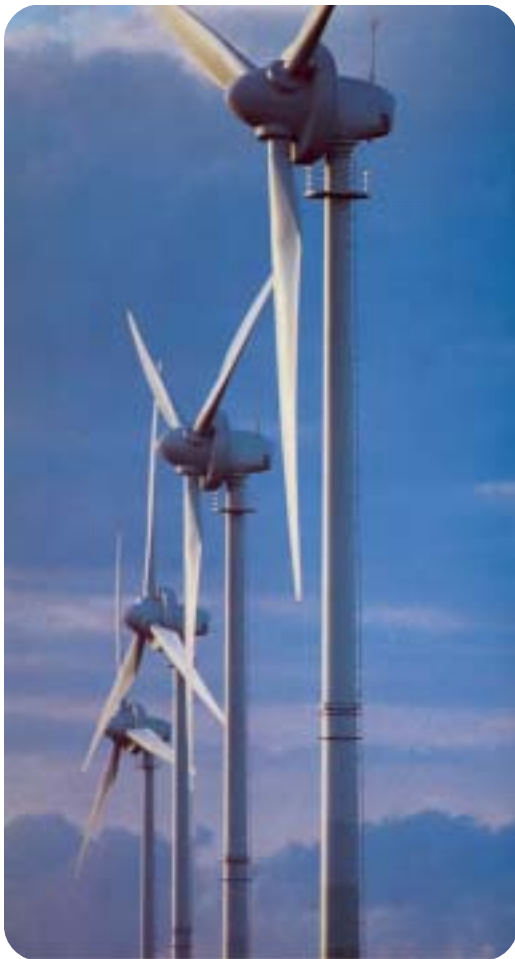
In power generation
