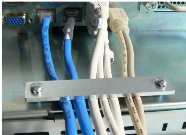
Cable Securing Bar Installed
