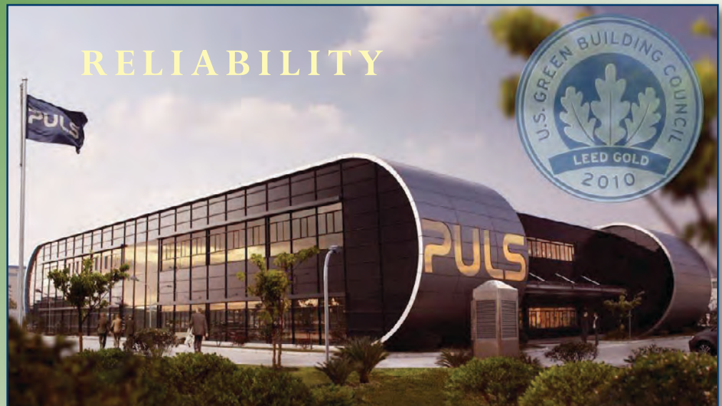
PULS Green Award Winning Plant in China
