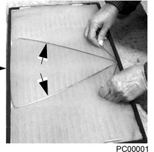
8. Install each filter frame to the bonnet on top of the cabinet.
