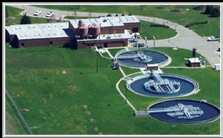
Clinton Reservoir Treatment Plant
